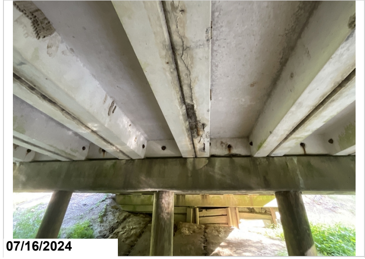
Span 1 unit 5 left leg spall 8LF CS3 at bent 2.
