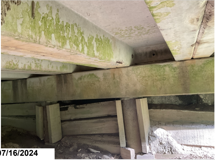
Span 2 unit 6 left leg spall 2LF CS3 at bent 3.
