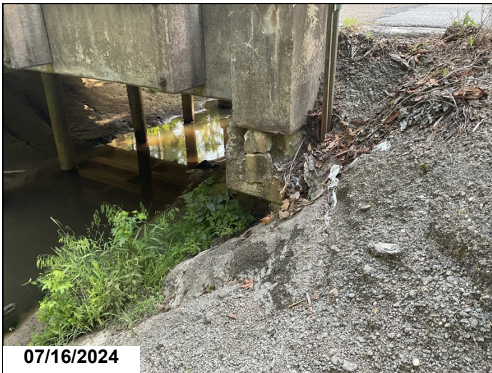
Bent 1 left side 2LF spall CS3
